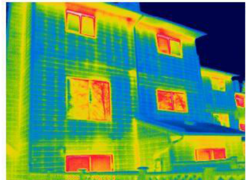
Infrared image of thermal bridging at studs, assembly interfaces, inside and outside building corners
